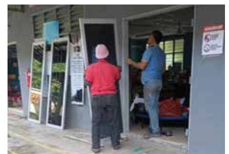
The doors of the school offices being replaced with new sets.
